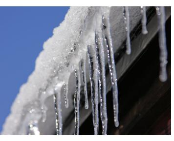
ICE BUILD UP IN DRAINS AND GUTTERS CAN RESULT IN WATER TO BE FORCED BACK UNDER YOUR ROOF CAUSING DAMAGE.
